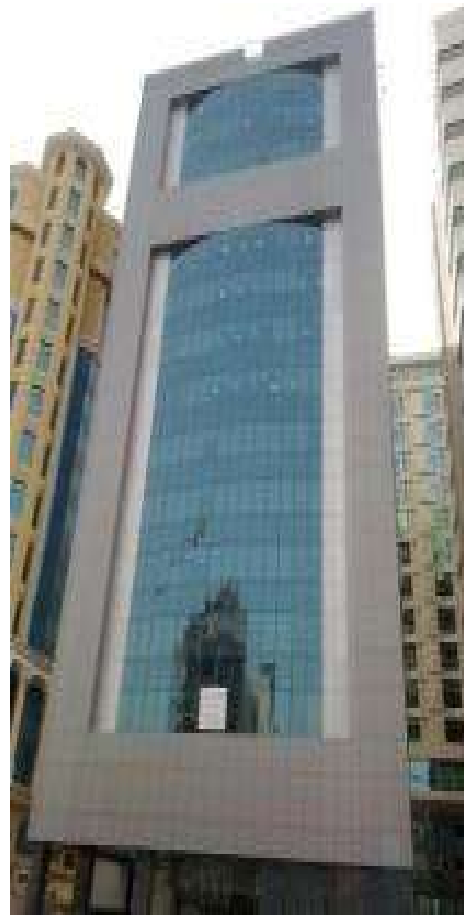
Jassim Tower at Old Salata Project Management
