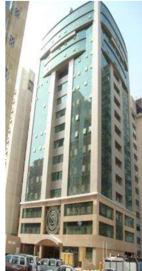
Hleyton Tower at Old Salata Project Management
