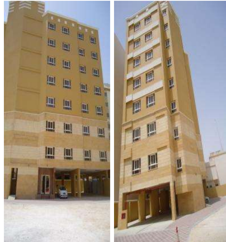
G+7 Hotel Apartment at Bin Mahmoud Construction, Completion & Maintenance
